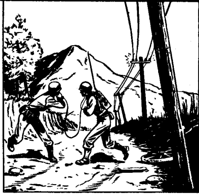
HIGH TENSION LINES
